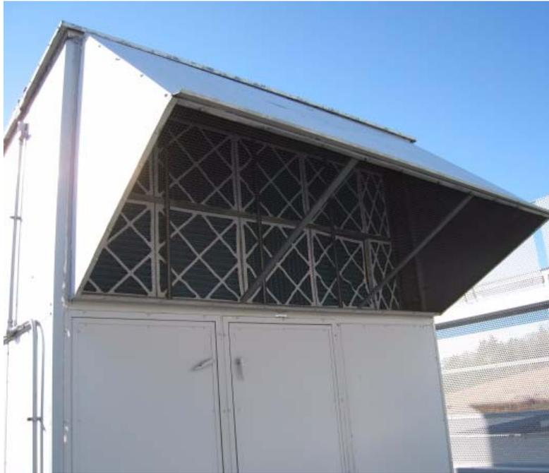
**Fresh Air Intake and Pleated Filter Bank for Rooftop AHU**
