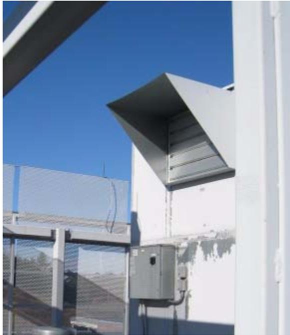
**Exhaust Vent of Rooftop Air Handling Unit Shut to Provide 100% Recycled Air**
