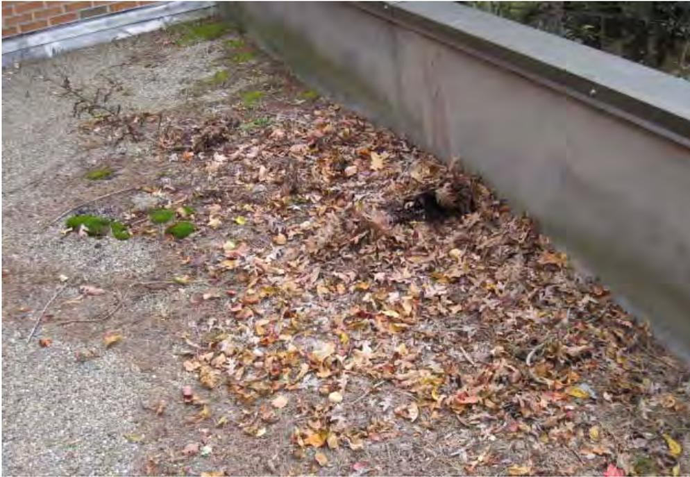
**Accumulated Leaves, Moss and Plant Debris on Roof**
