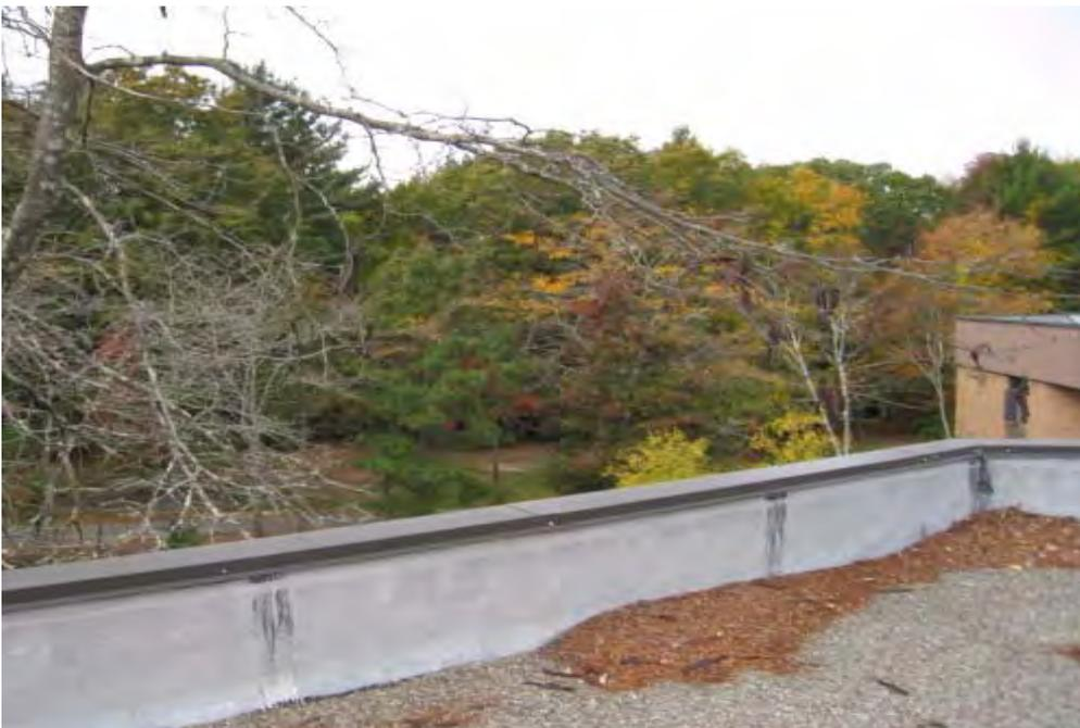
**Overhanging Branches and Accumulated Plant Debris on Roof**
