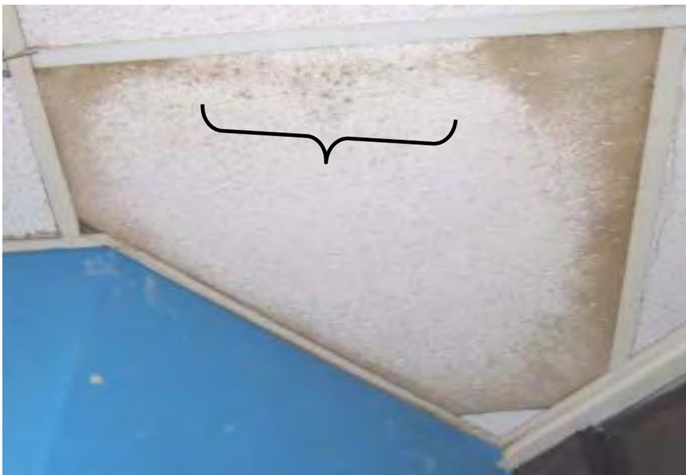
**Water Damaged Ceiling Tile in Classroom, Noted Area Indicates Possible Mold Growth**
