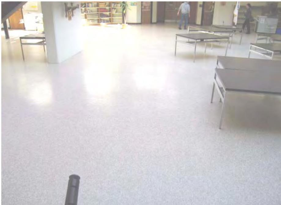
**Carpeting Removed in Lower Level Media Center Replaced with Tile**
