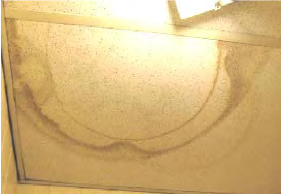
**Water Damaged Ceiling Tile in Classroom/Restroom**
