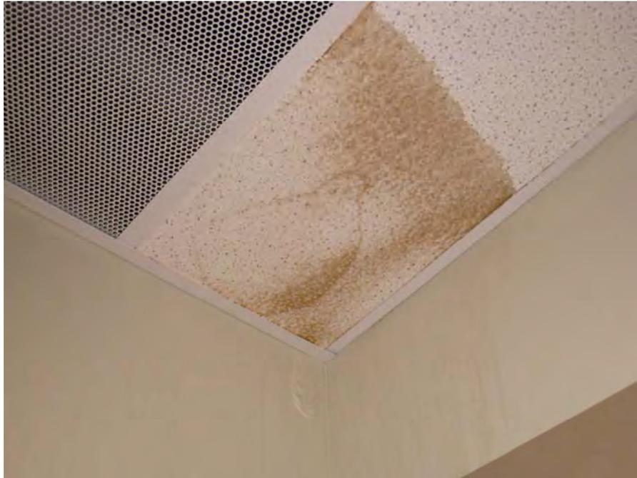
**Water-damaged ceiling tile and bubbled/stained wall paint in area 243**
