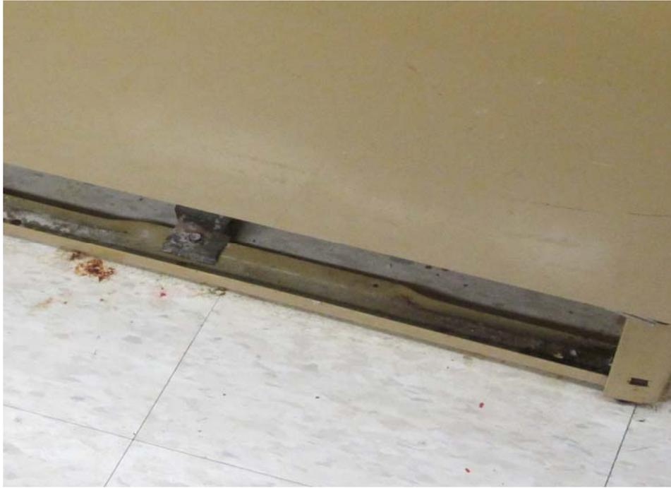
**Missing drip pan under the refrigerator**
