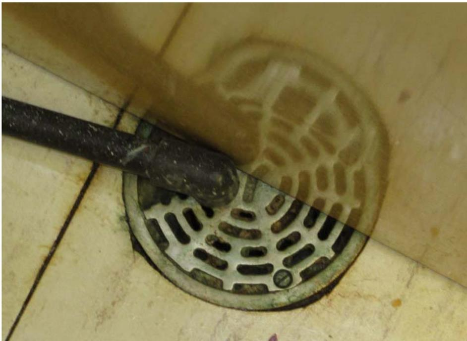
**Floor drain in kitchen (note: partially obstructed by the refrigerator)**
