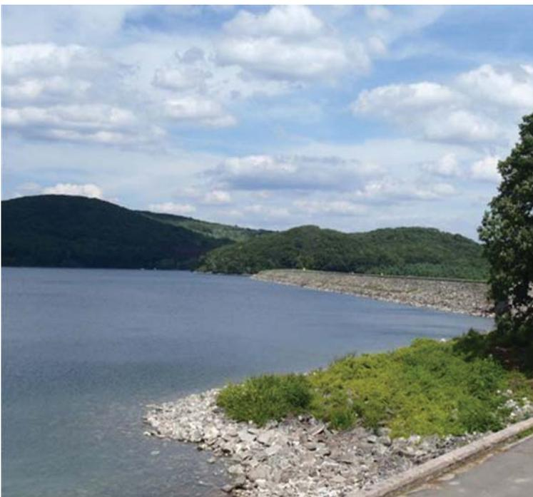
Just to the east of the Administration Complex one can see the Winsor Dam, an earthen structure with stone facing that holds back the 412 billion gallon Quabbin Reservoir (left). The Quabbin Observation Tower (right) situated at the summit of Great Quabbin Hill, is an 84' tower that was completed in 1941 for use as a fire watch tower as well as for public viewing. Accessed via Rt. 9, recent rehabilitation has made it ready for the fall "leaf peeping" season.
