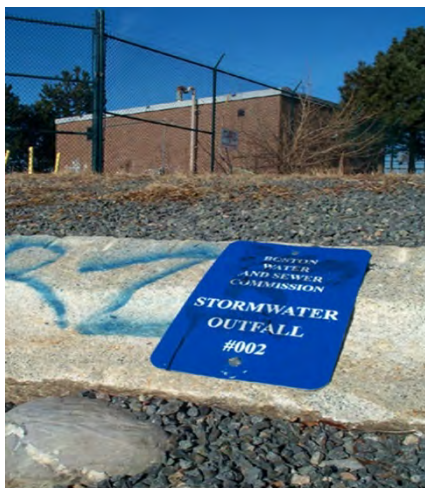
MWRA decommissioned its Constitution Beach CSO Facility after CSO flows were eliminated by BWSC sewer separation.
