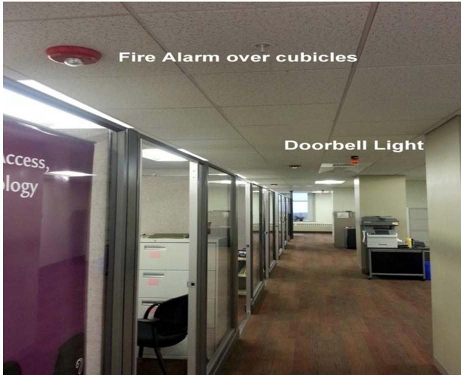
**Figure 1:** Hallway outside MCDHH showing the placement of fire alarm over cubicles and doorbell lights
