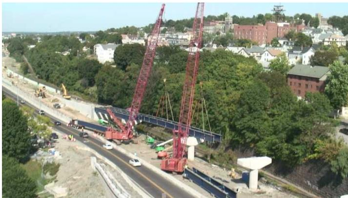
*Structural steel being set in place for the new on-ramp from I-195 WB to Route 79 NB.*
