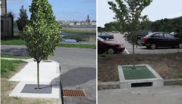
Tree filter with attached catch basin (left) or curb inlet (right).
