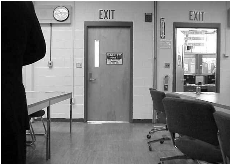
Space Beneath Classroom Door Adjacent To Metal Shop
