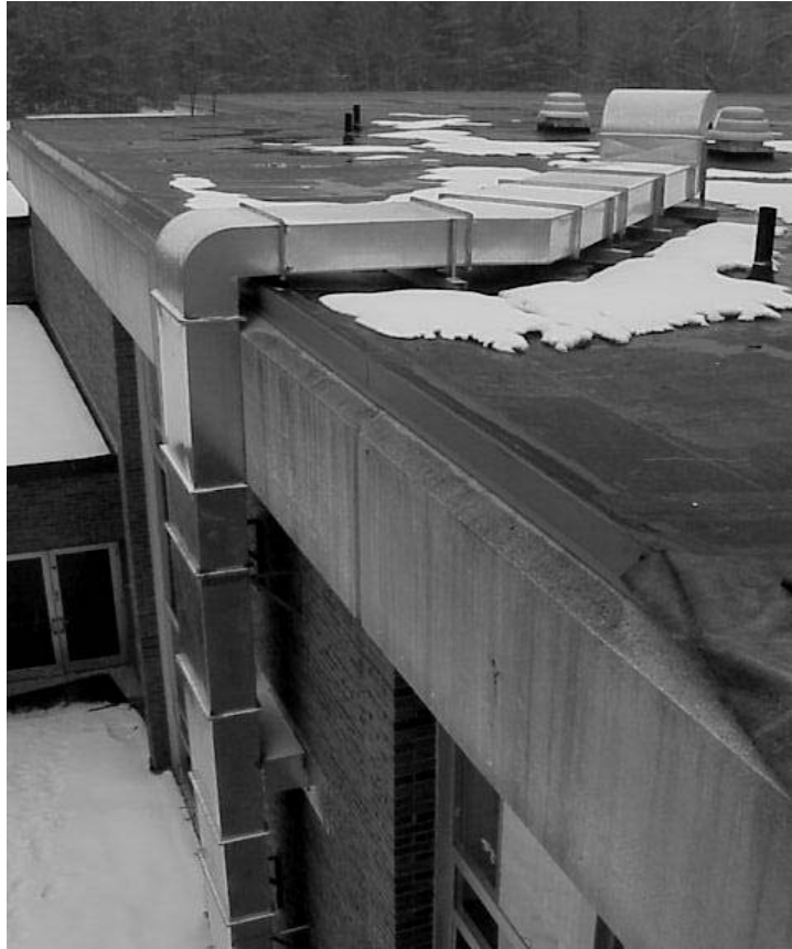
Ductwork Installed for Fresh Air Intakes of Classrooms 106, 108, 210 and 212
