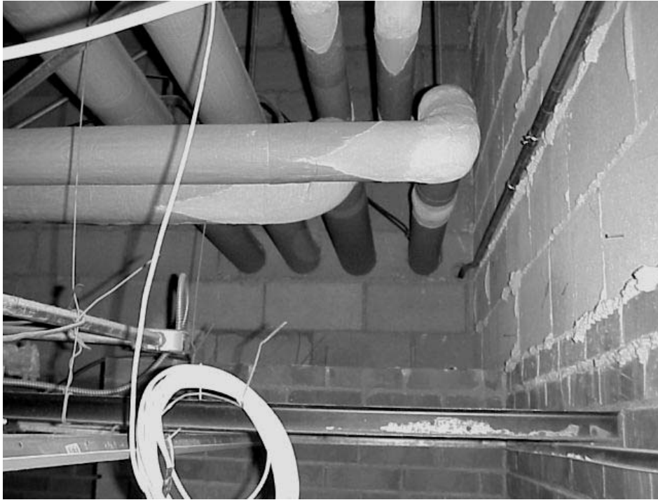
Plenum above Suspended Ceiling Pictured through Missing Ceiling Tiles
