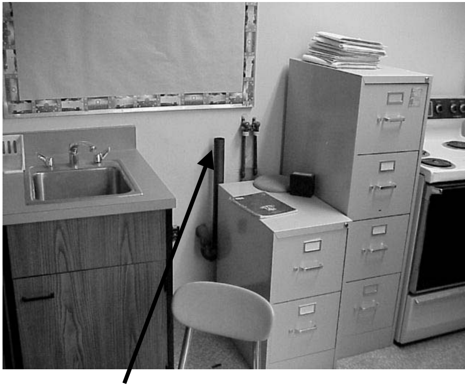
Open Clothes Washer Drainpipe in Classroom 224
