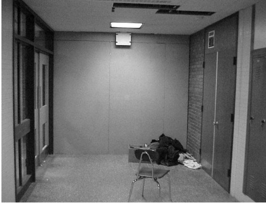
Temporary Wall Sealing Renovations From Occupied Area Of School
