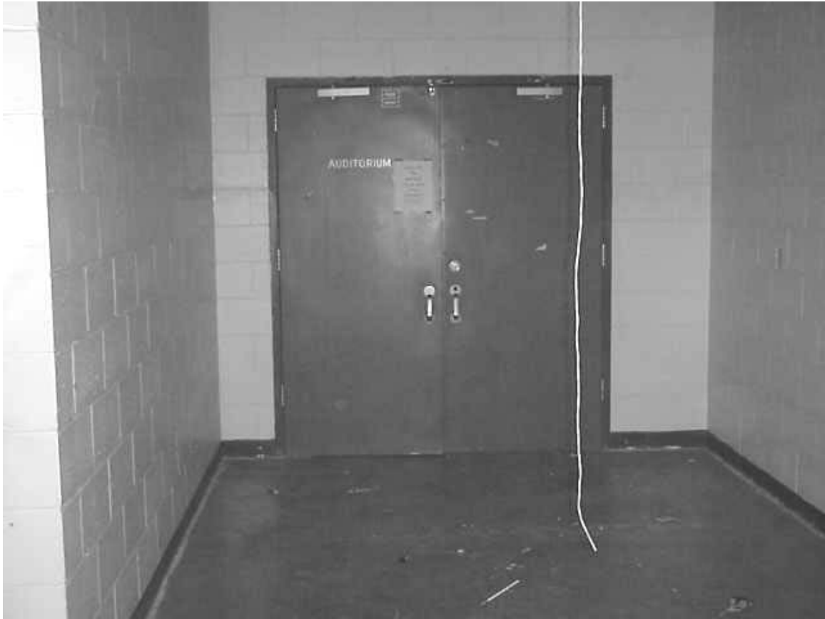
Auditorium Doors Noted in Construction Zone on 2nd Floor of D-wing
