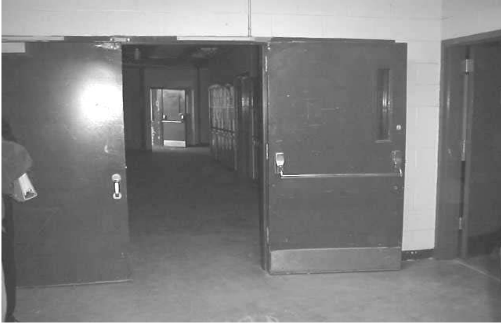
Interior Doors Located In Construction Zone
