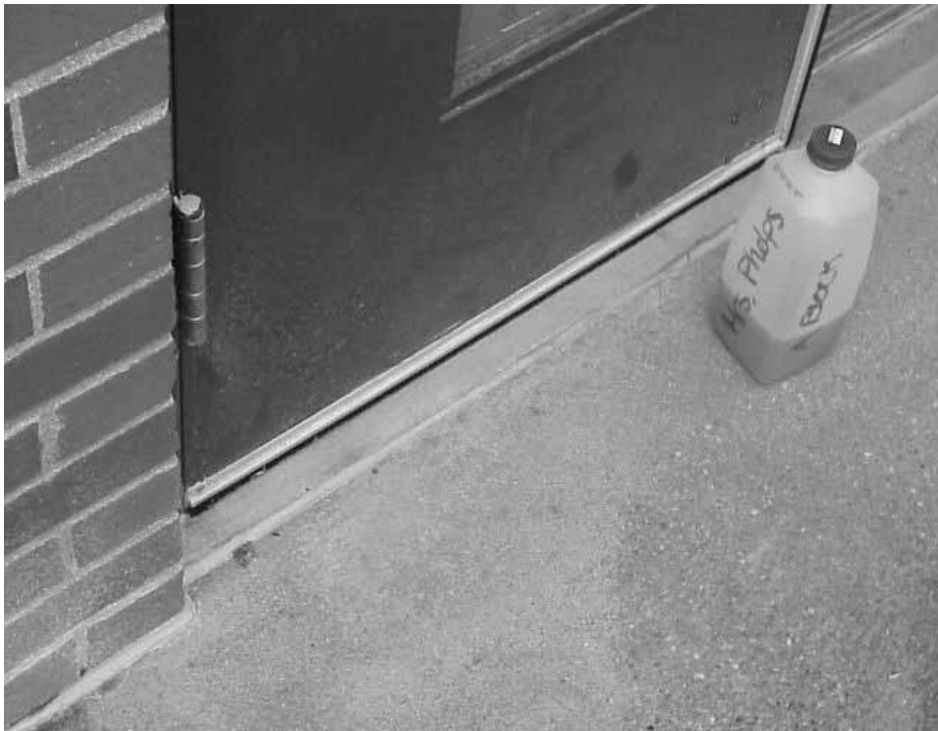
Sealant Applied To Door Threshold, Concrete Slab and Exterior Wall Junction
