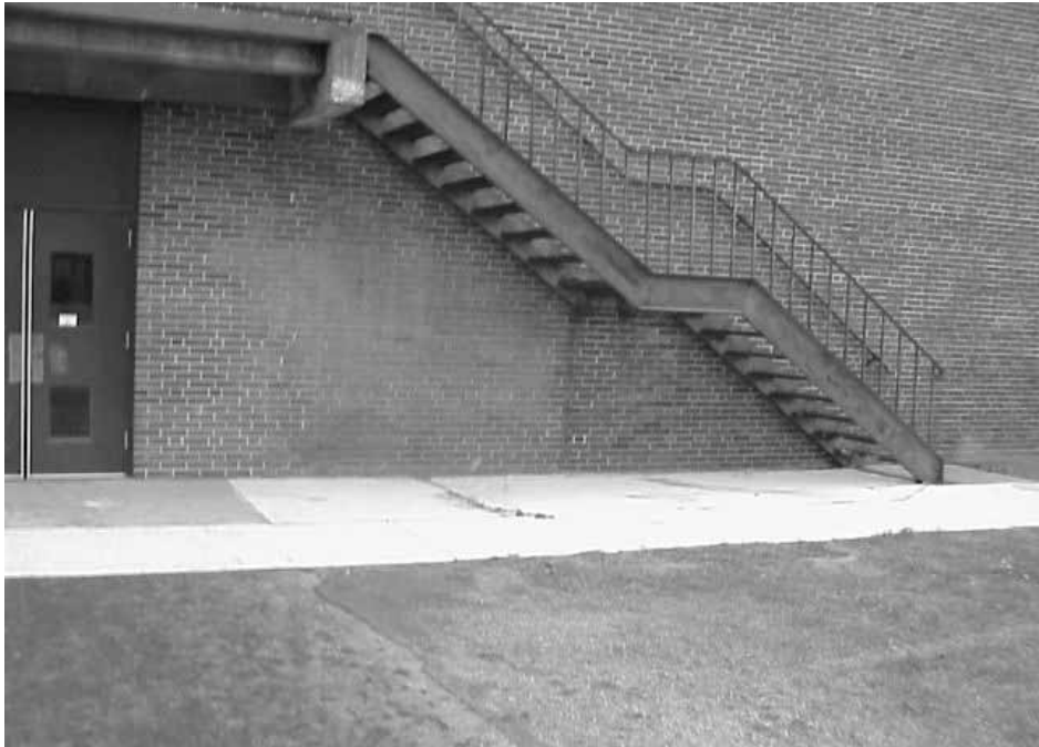
Concrete Pad Installed beneath the Concrete Platform
