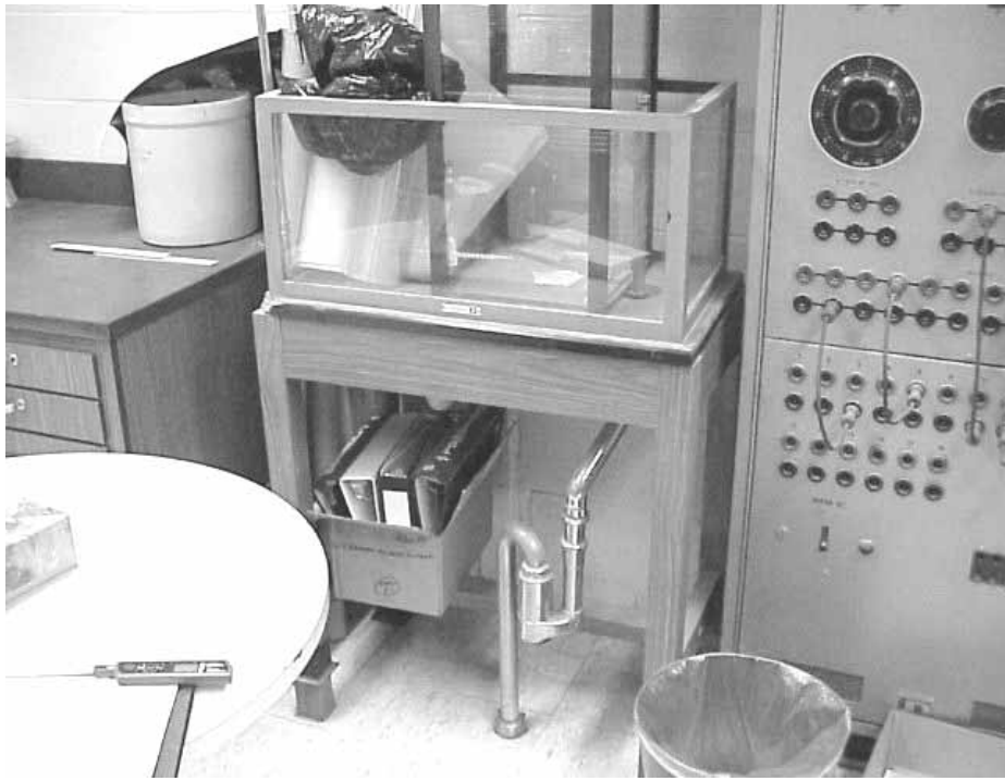
Aquarium-Like Equipment Attached To Drains with Traps
