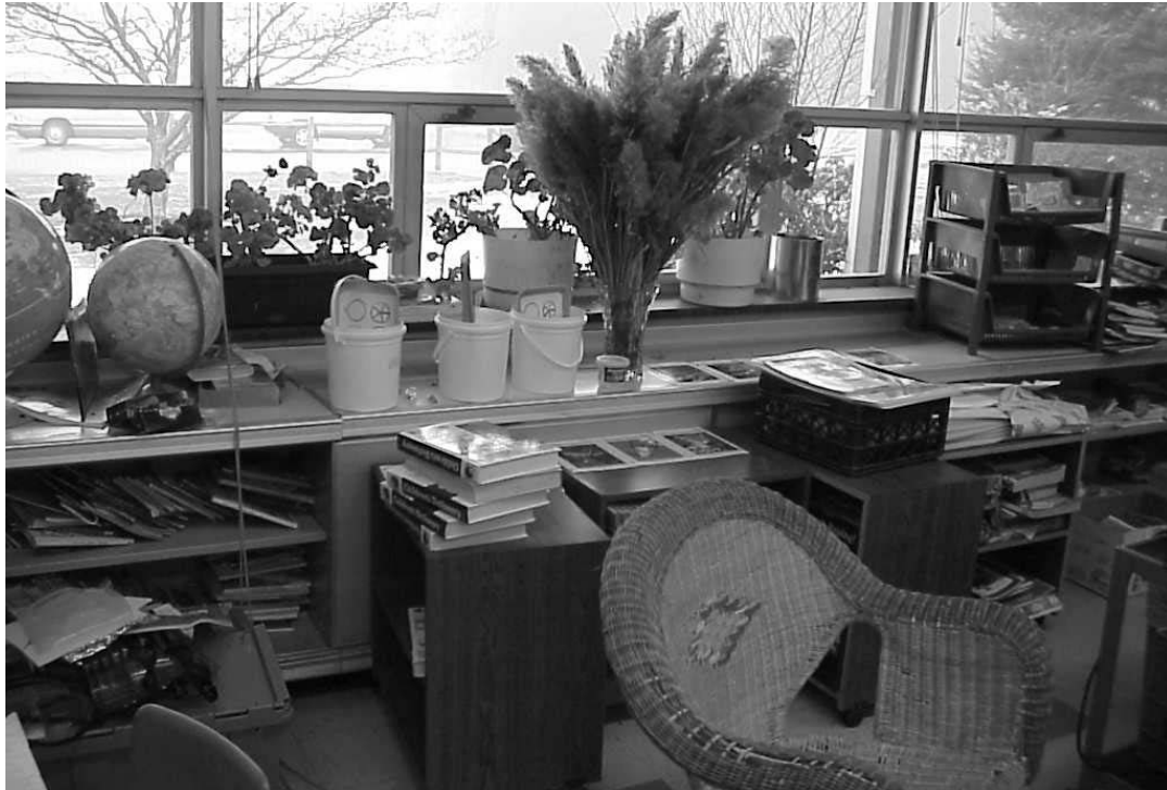
Plants over Air Diffusers of This Classroom's Univent
