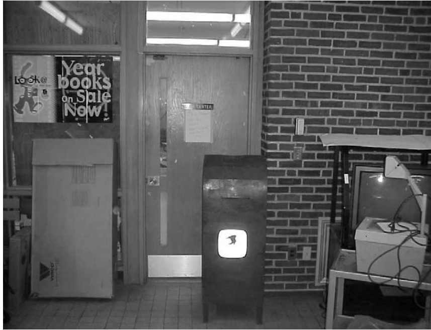
Unsealed Door to Library under Renovation
