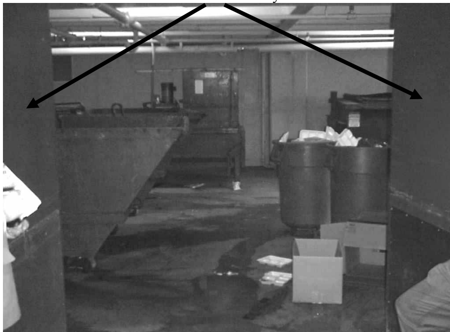
Trash Dumpster Store Room
