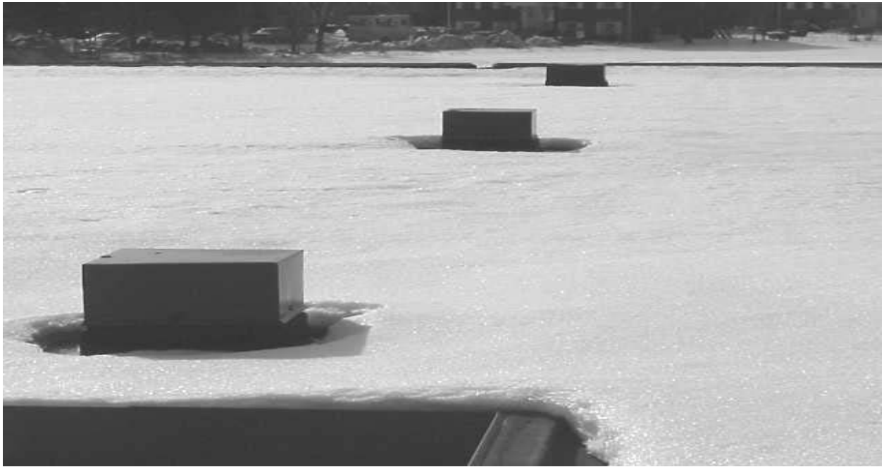
Former Exhaust Ventilation Ducts Sealed with Sheet-Metal
