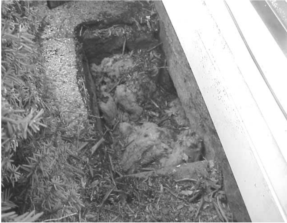
Exterior Shot of Window Casing Sealed with Fiberglass Insulation
