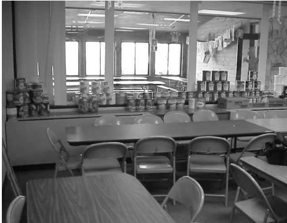
Interior View of Kitchen/Cafeteria, Univalent Fresh Air Intakes Sealed Indoors Are Located below Windows
