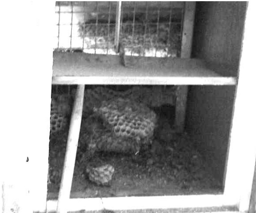
Wasp Nests in Exhaust Vent
