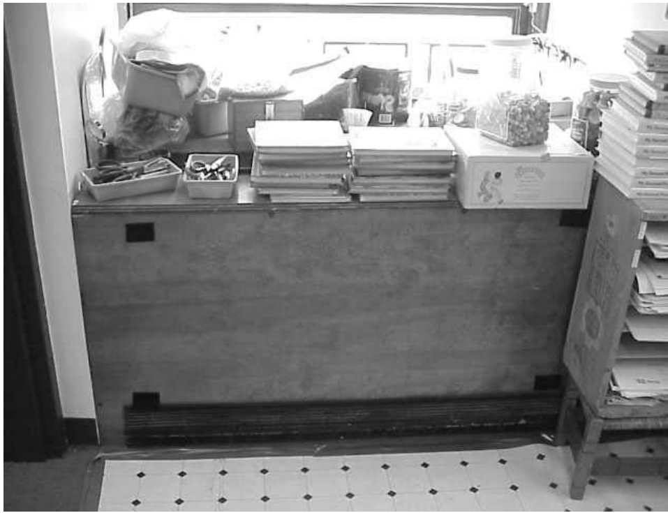
Univent in Wooden Casing
