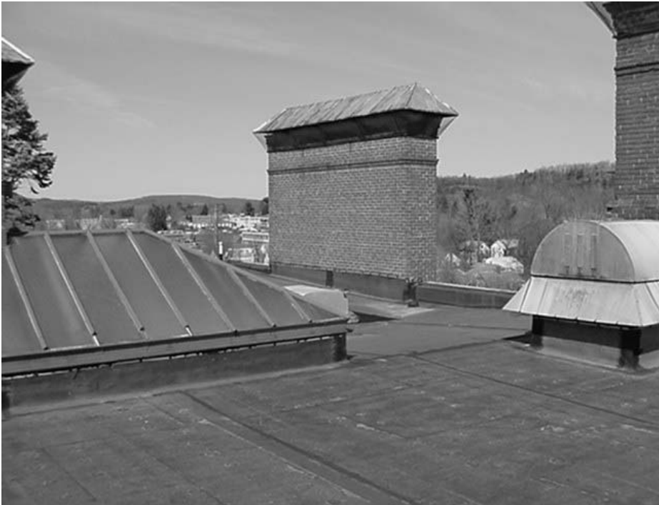
Capped Air Shaft on North Wing Roof
