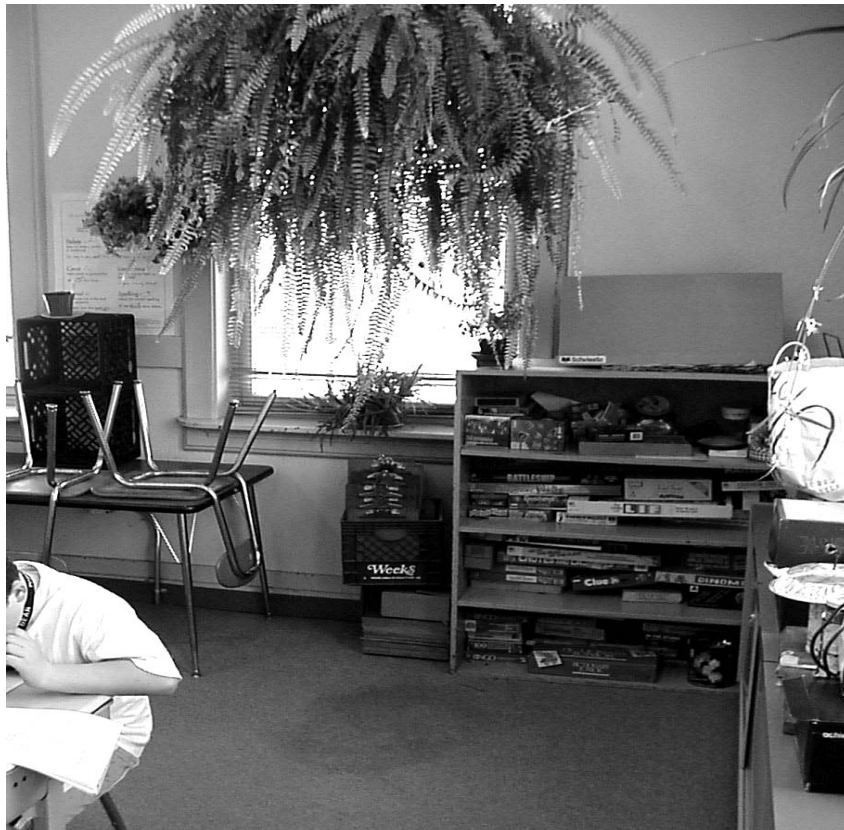
Plant in Classroom, Note Water Stain on Carpet beneath Plant
