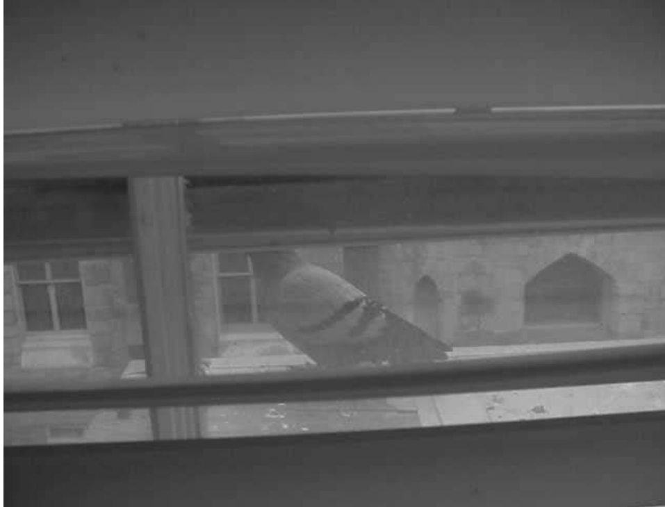
View from Indoors of Pigeon on Top of the DPW Engineer's Office Window-Mounted Air Conditioner Casings
