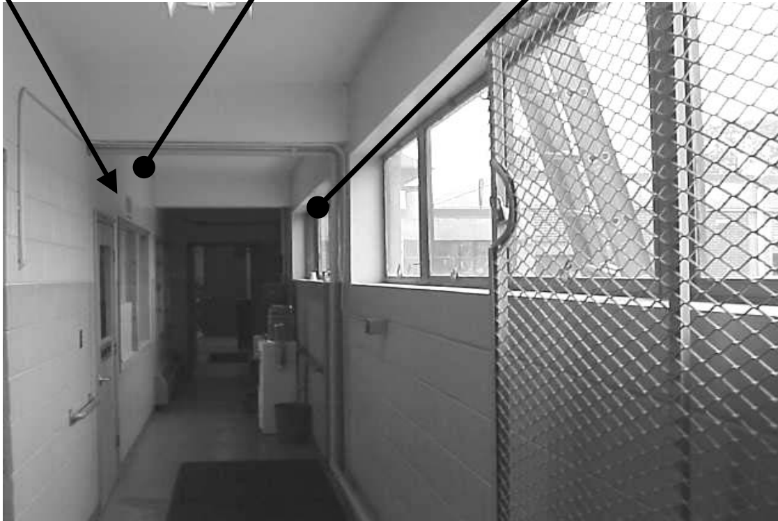
Openable Windows on Exterior Wall of Water Department Administration Building Note Windows are Separated from Occupied Billing Area by Interior Wall
