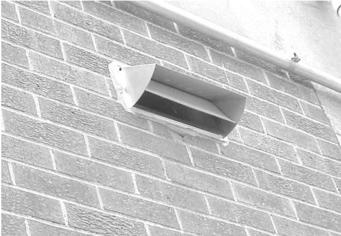
Exhaust Ductwork for Conference Room Noted on West Exterior Wall
