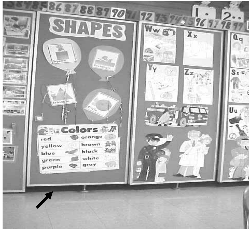
Doors of Classroom Coat Closets: Note Doors are Undercut to Facilitate Exhaust Ventilation
