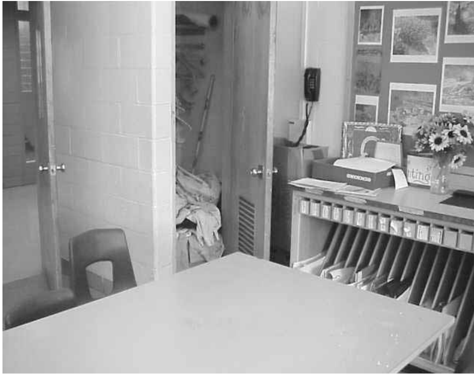
Piled Materials Blocking Closet Passive Door Vent
