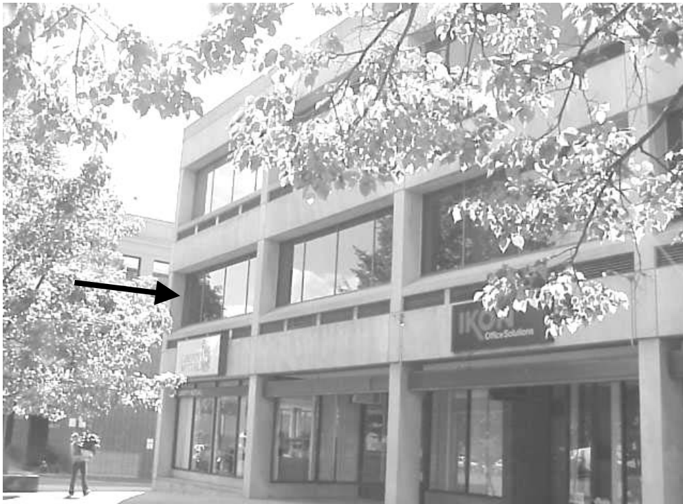
DOR CSE Office Located on Second Floor of Building
