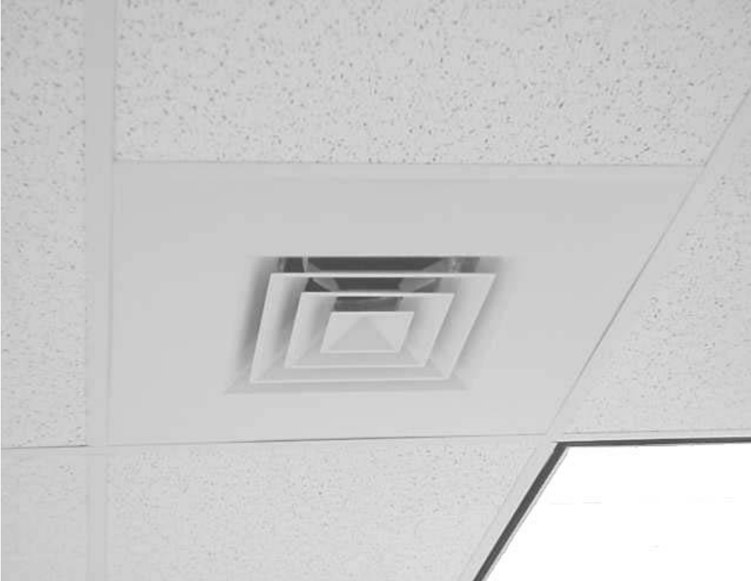
Ceiling-Mounted Multi-directional Air Diffuser
