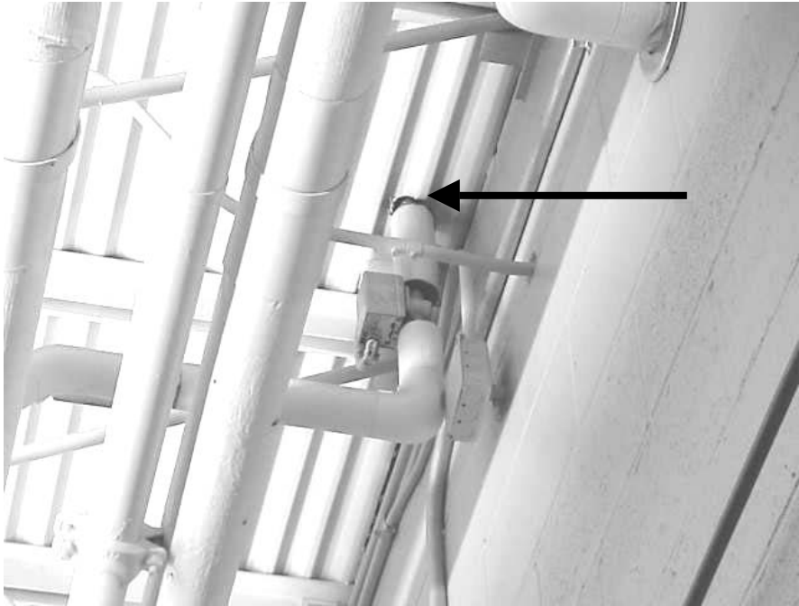
Utility Hole in Engine Bay Ceiling Decking
