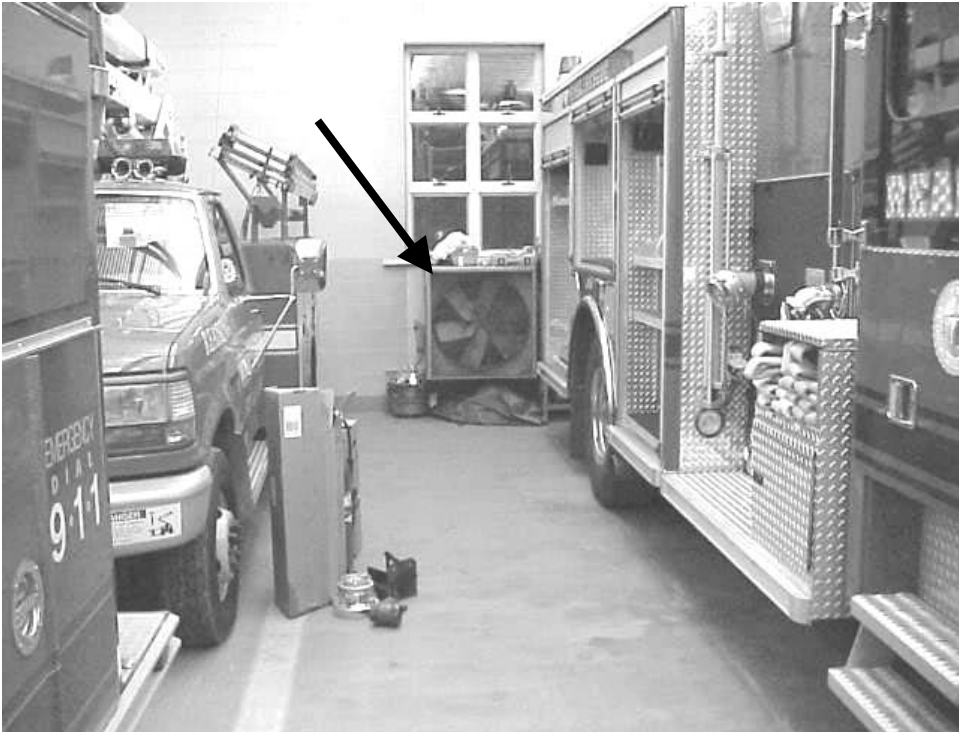
Floor Exhaust Fan in Engine Bays
