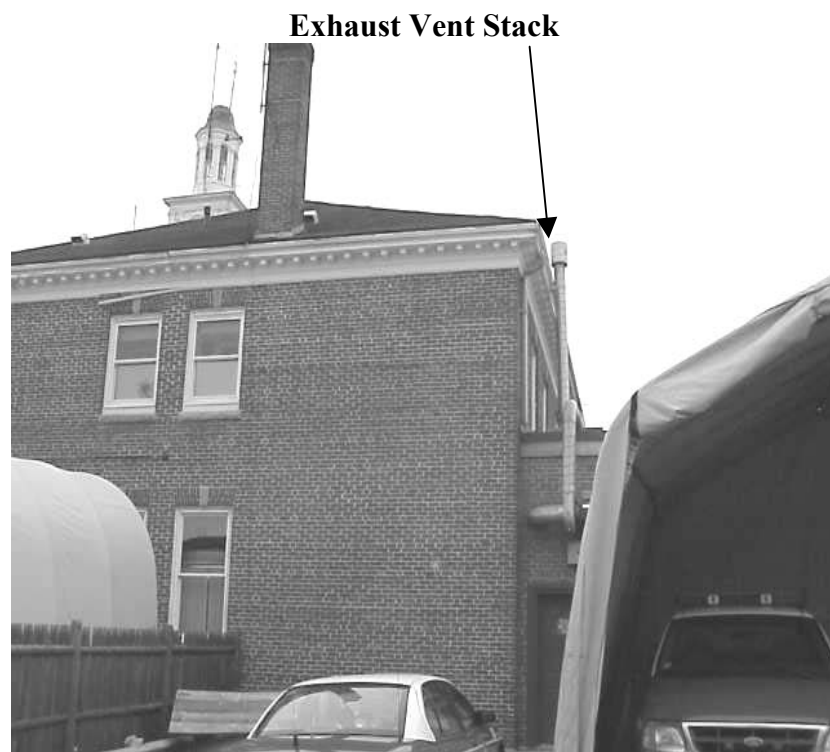
Vehicle Exhaust Vent (40 West Central Street Firehouse, Franklin, MA), Note the Position and Height of Vent away from Windows at rear of Building
