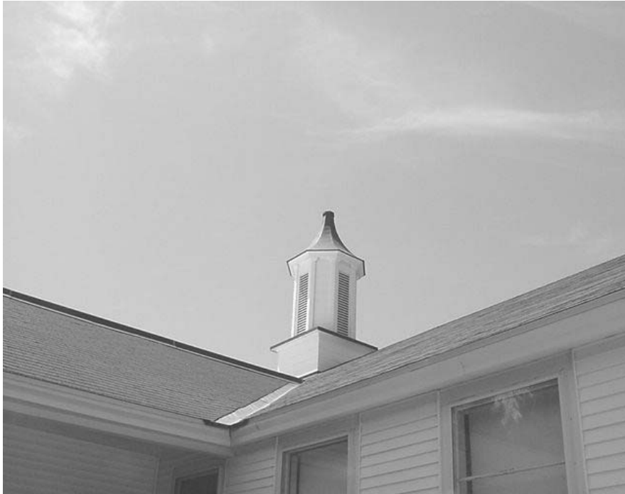
Rooftop Cupola That May Contain Exhaust Vent Terminus
