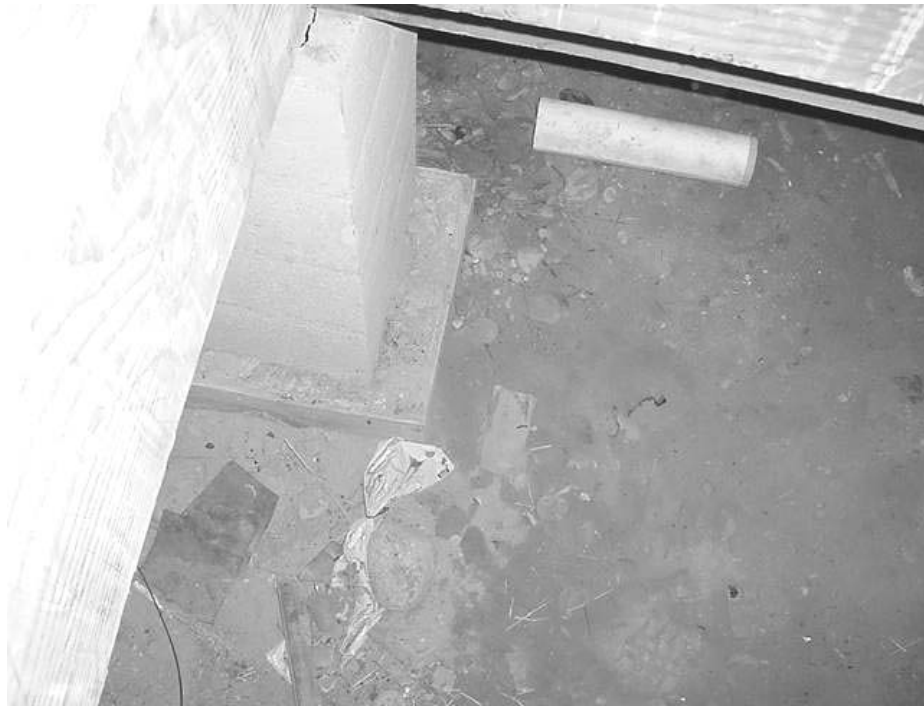
Floor Of Crawlspace beneath 1947 Wing
