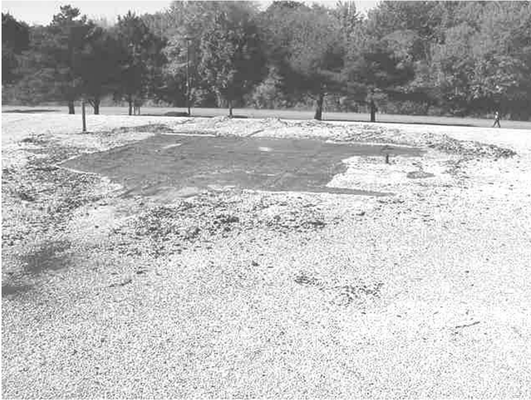
Area on Roof Cleared Away to Isolate and Repair Leak
