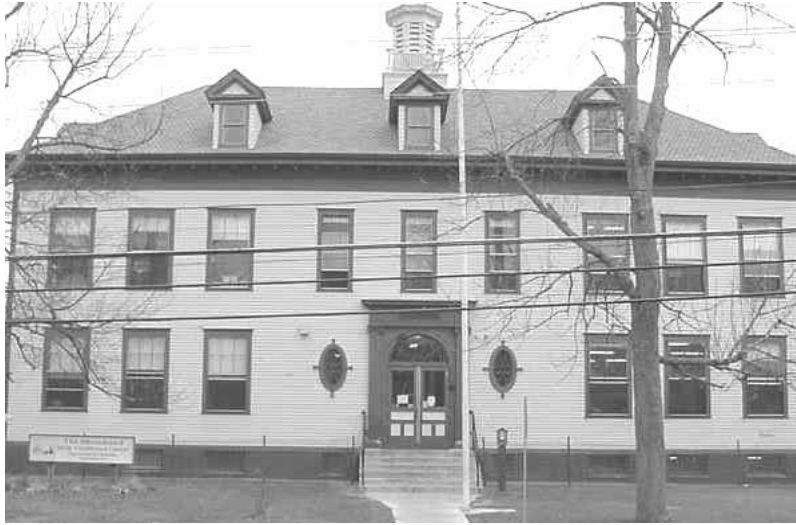
The Original School Building, Constructed In 1870
