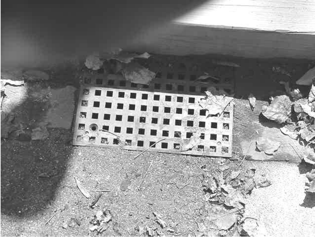
French Drain Installed to Prevent Flooding of Basement
