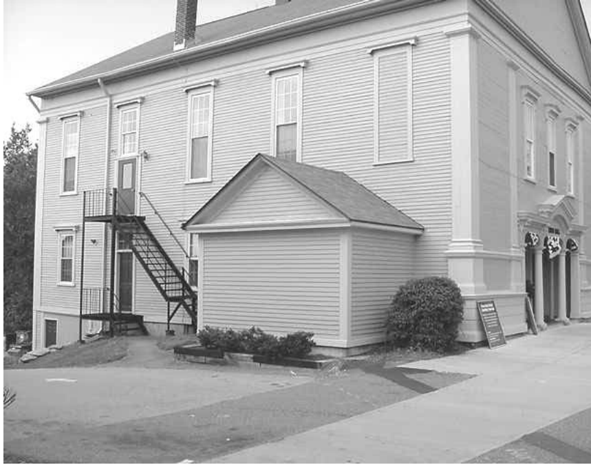
The Addition, Note Shrubbery and Lack of Gutters/Downspout of Roof Edge
