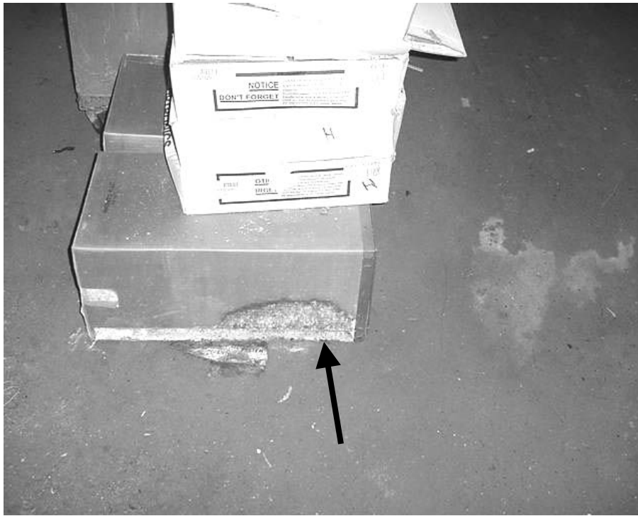
Basement with Dirt Floor, Note Mold Colony on Box
