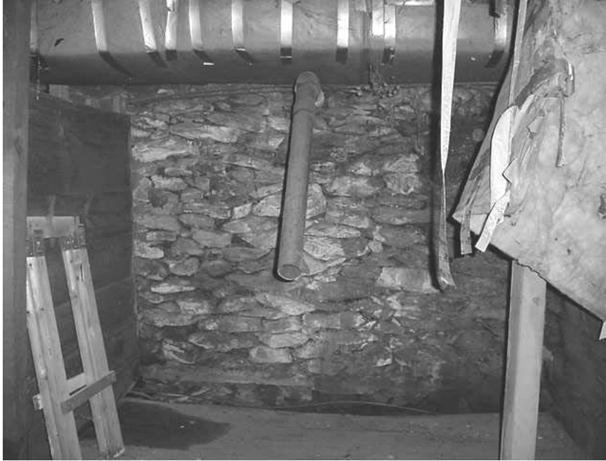
Open Pipe in Basement
