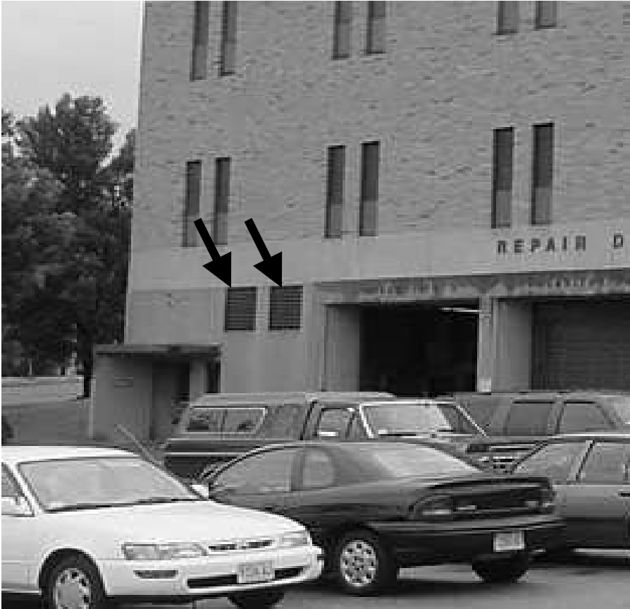
Ventilation System for Repair Shop
