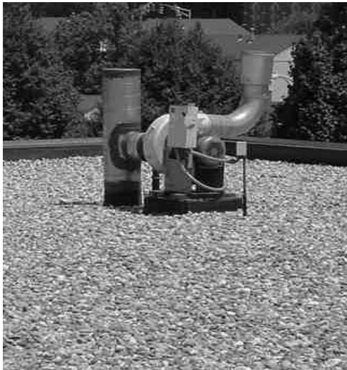
Special Design Vehicle Exhaust Removal System for Operating Fire Engines and Related Vehicles
