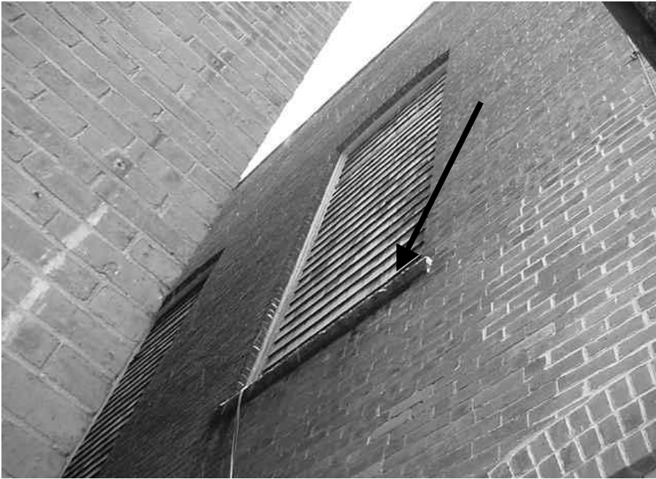
Flat Ledges along Building Exterior
