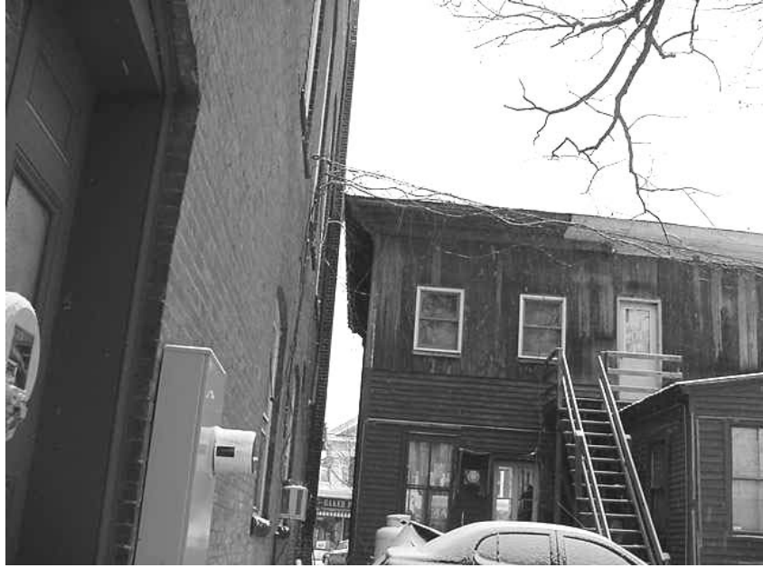
Peaked Roof Building Immediately Adjacent to the Town Hall
