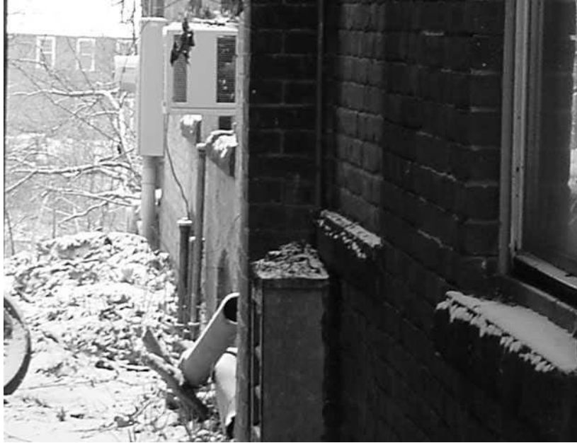
Dirt Floor Alleyway
