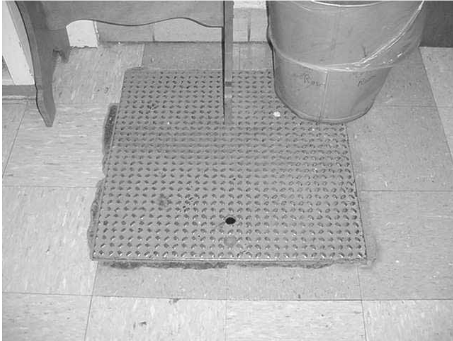
Crawlspace access door
