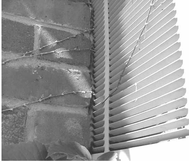
Air Conditioner Cabinet with Fixed Louvers Inside Building Envelope
