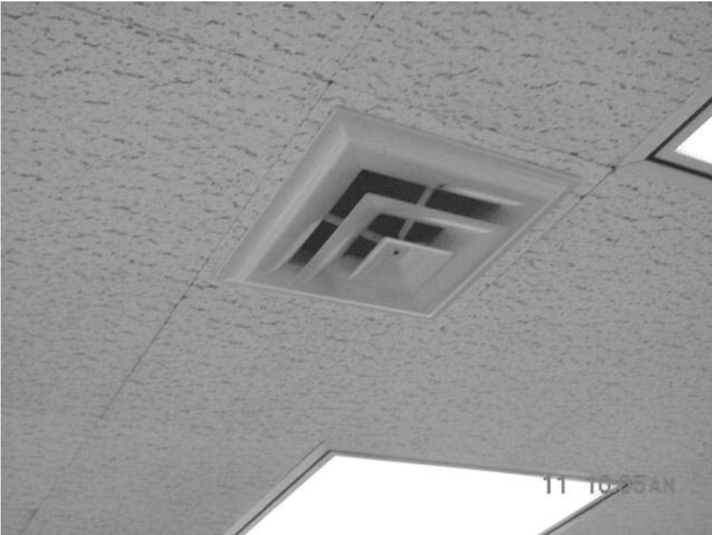
Ceiling-Mounted Air Diffuser
