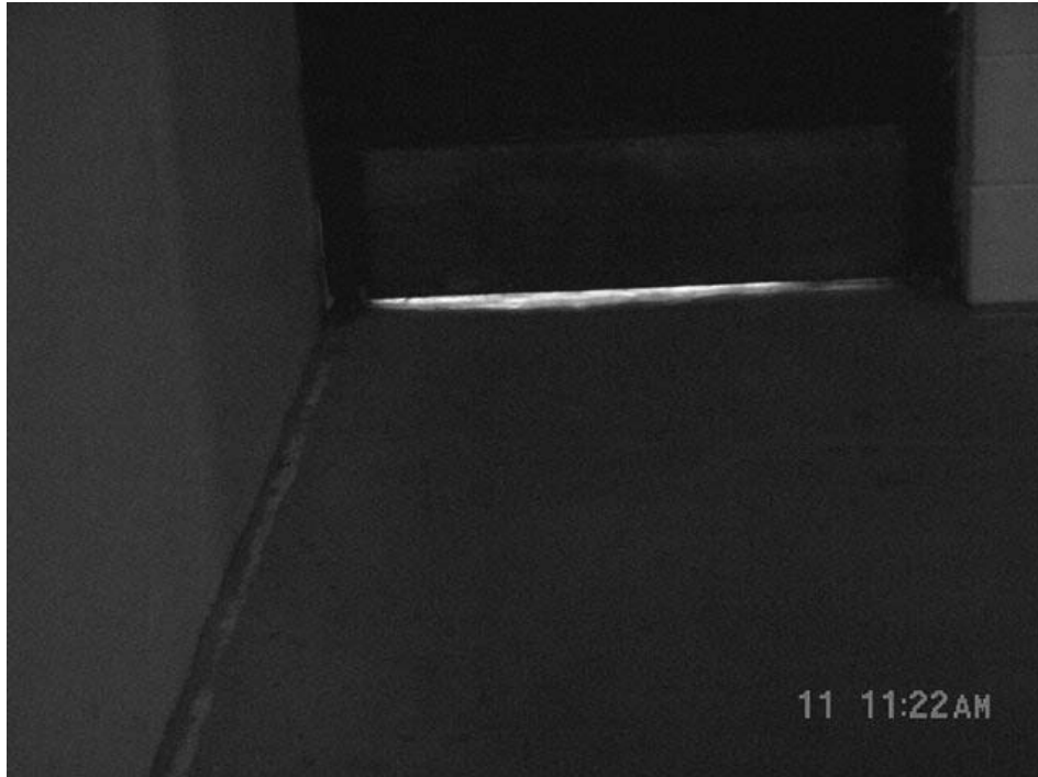
Light Penetrating beneath Parking Garage Door (when closed)
