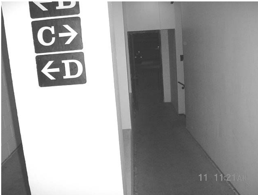
Hallway Accessing the Parking Garage, Note Door to Garage Propped Open
