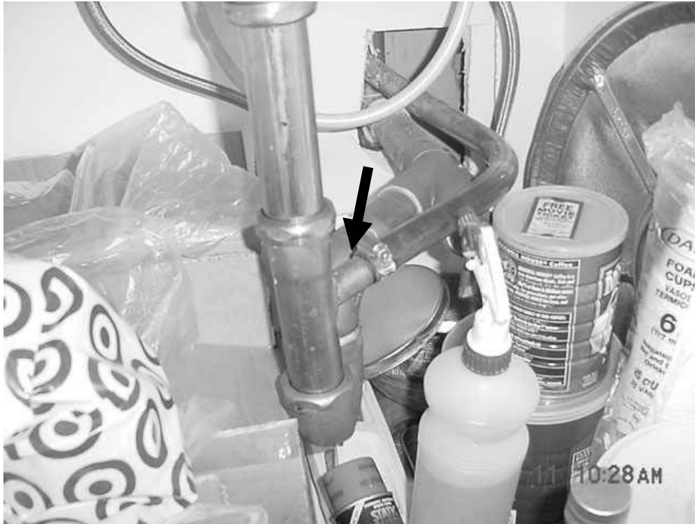
Terminus of Hose from Temporary Drainage System in Previous Picture
