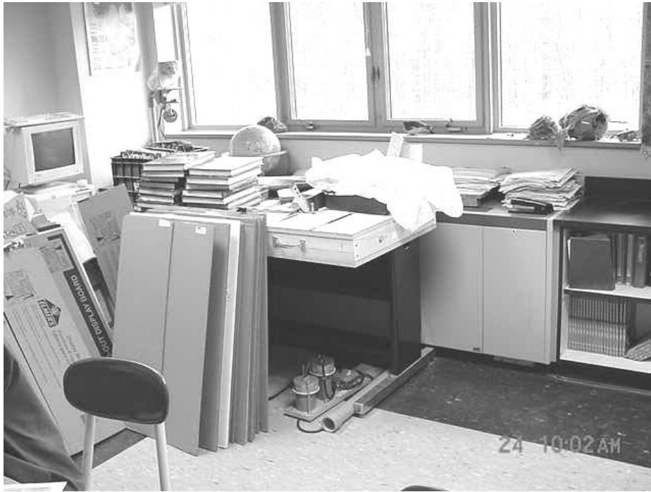
Classroom Unit Obstructed by Various Materials on and in front of Unit
