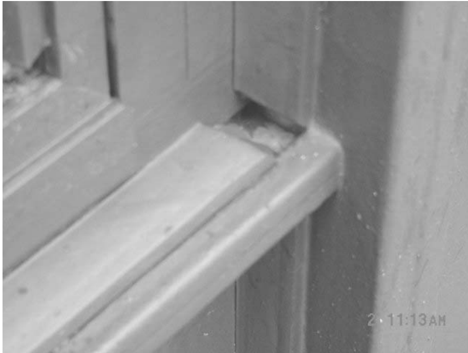
Spaces between Exterior Wall Panels (see Picture 13 for Comparison)
