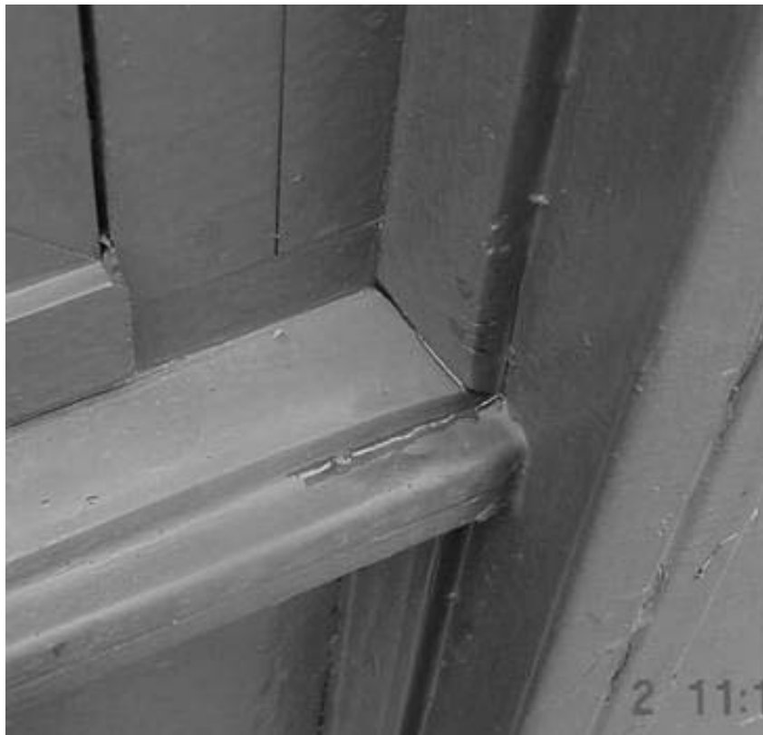
Exterior Wall Panel Sealed
