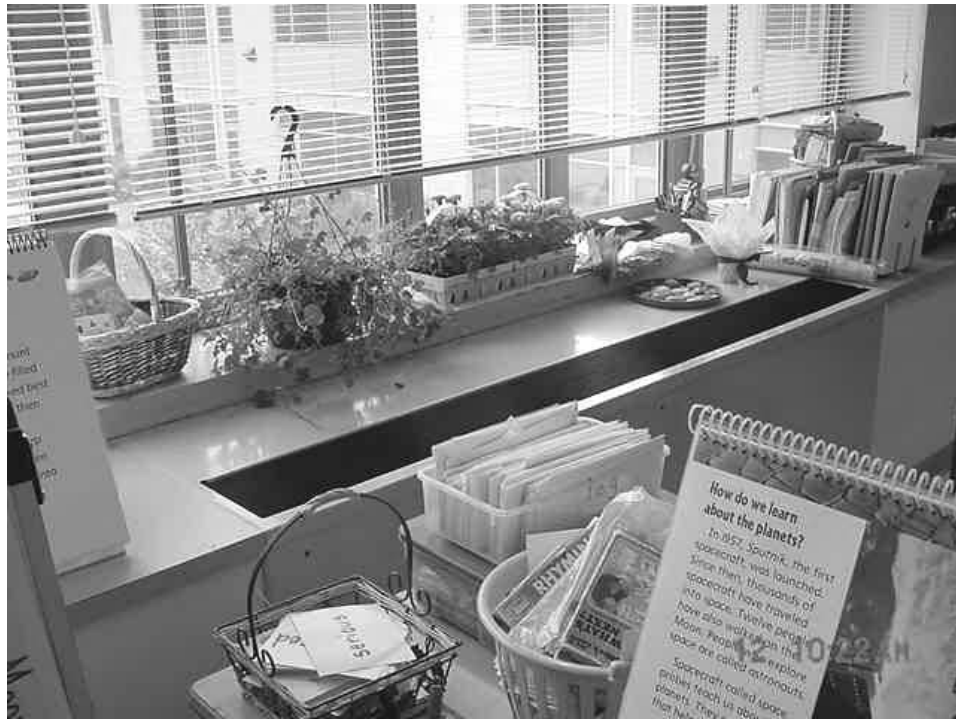
Plants near Univent Air Diffuser
