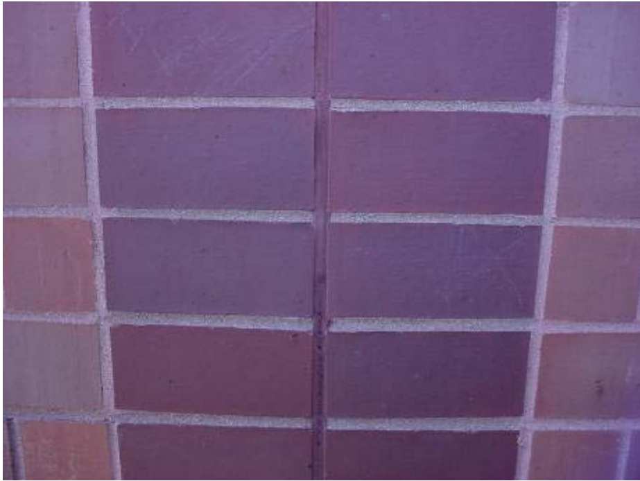
Sealed Expansion Joint
