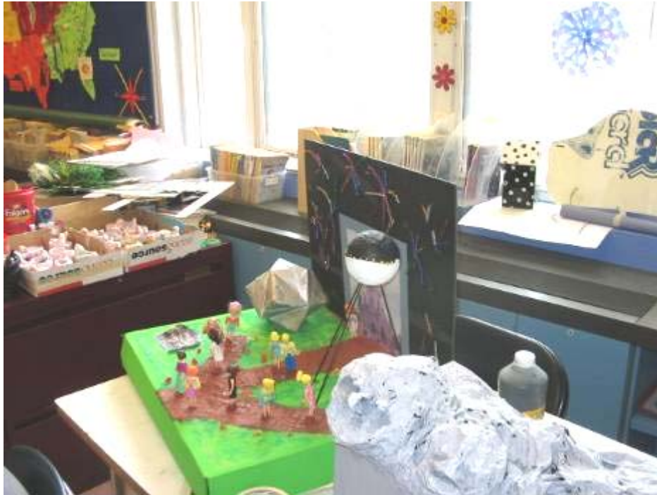
Univent Blocked by Furniture and Store Materials
