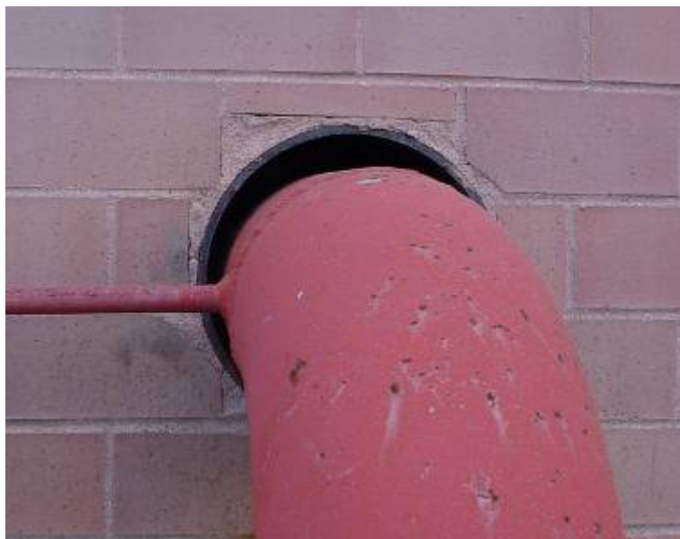
Spaces around Utility Hole
