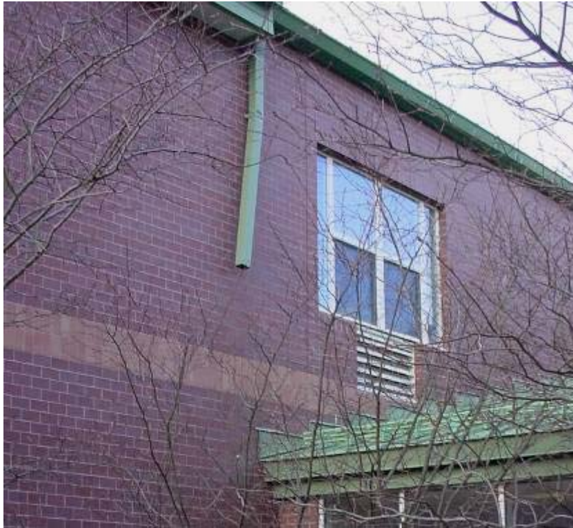
Missing/Damaged Downspout
