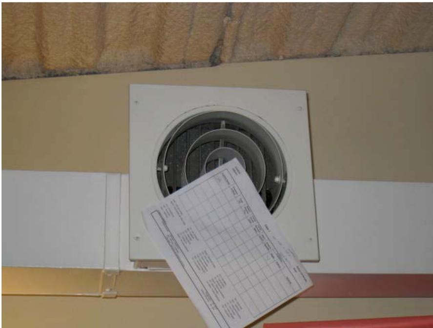
**Exhaust fan in common area, note paper shows draw of air into vent**
