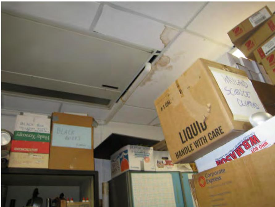
**Ceiling-mounted AHU, note water-damaged tiles and stored items**
