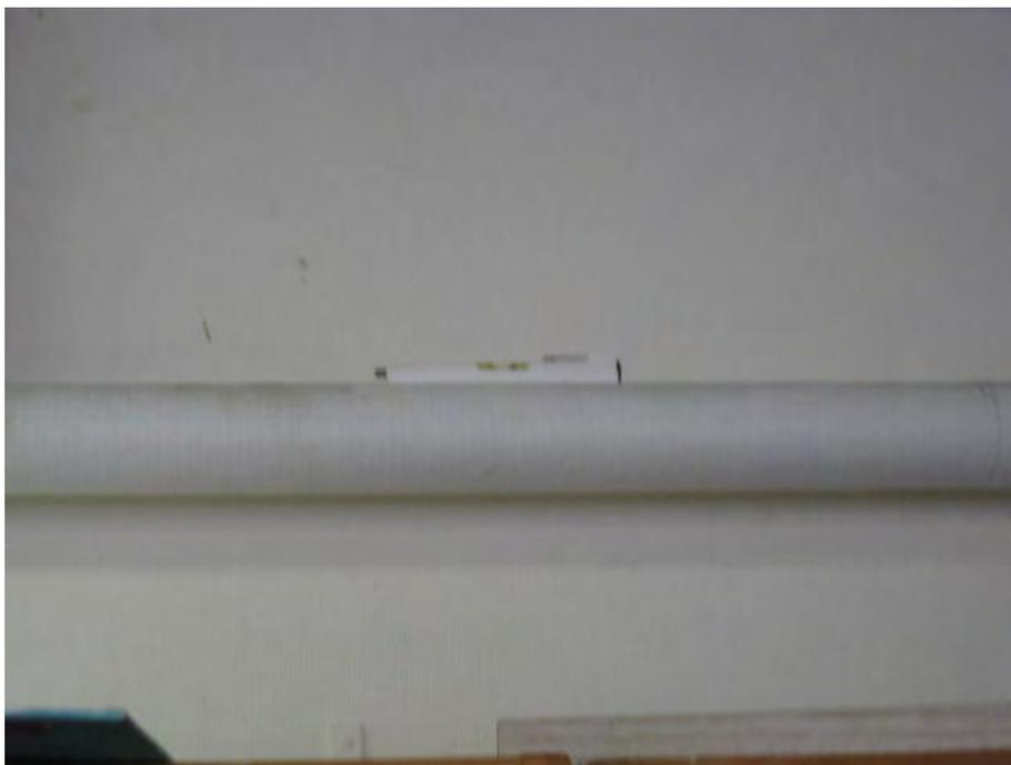
**Condensation Drain Pipe with Level, Indicates No Pitch to Pipe**
