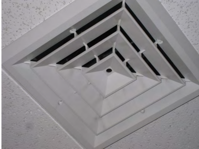
Typical Fresh Air Supply Diffuser
