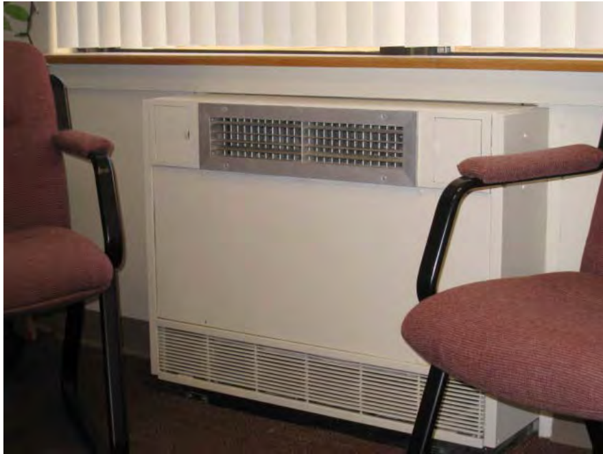
Typical Fan Coil Unit
