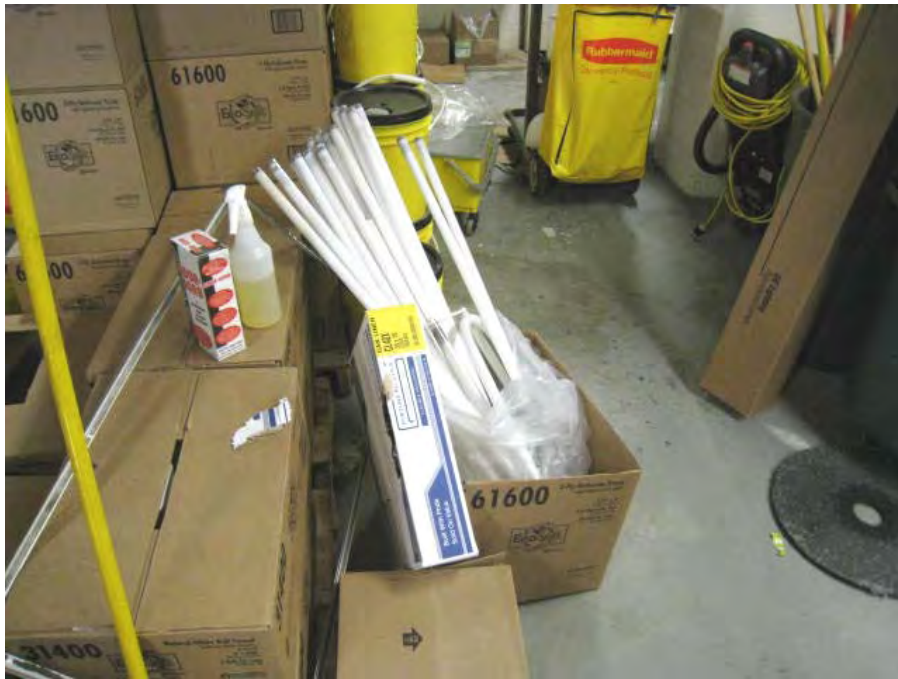
Freestanding fluorescent lights in storeroom
