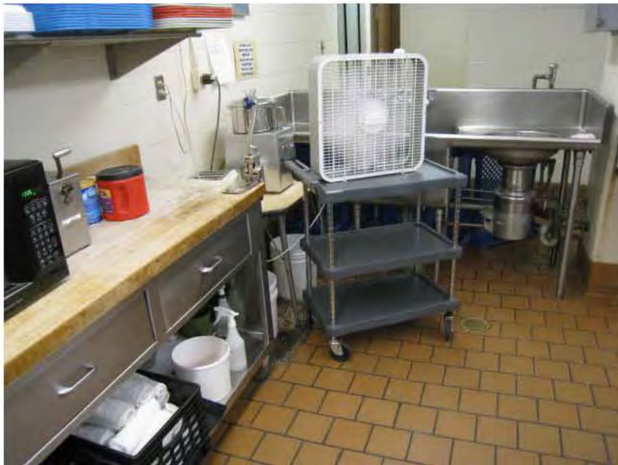
Portable fan in the kitchen
