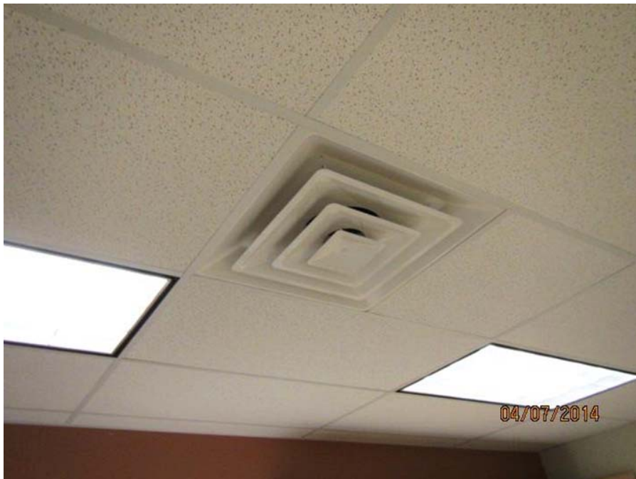
Typical supply diffuser
