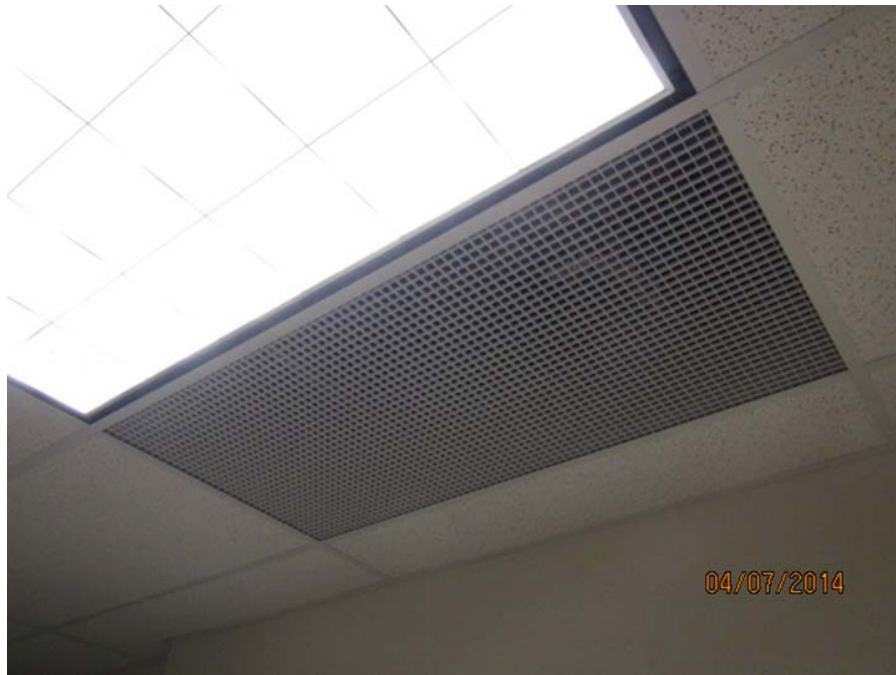
Typical exhaust grate
