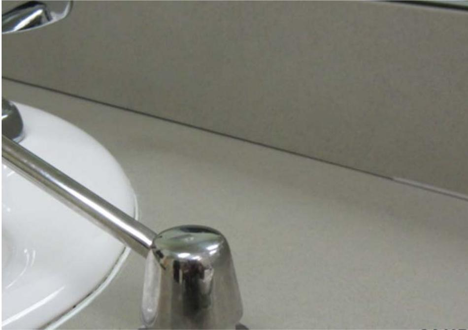
**Missing caulking in bathroom sink**
