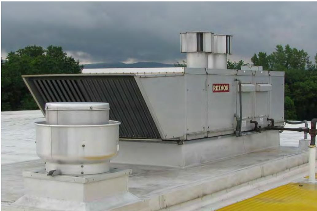
**Exhaust vent in close proximity to AHU fresh air intake**
