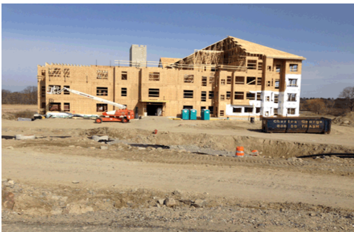
Residential Bldg. 1000, which is scheduled to be complete by September 1, 2013
